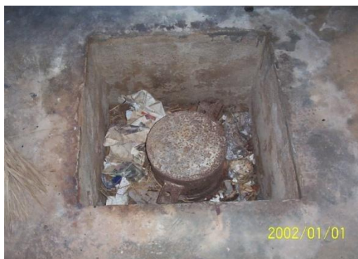
Fig. 17: The Kapasda Water Supply Scheme P.H.No-1, abandoned due to saline water intrusion, Contai, Purba Midnapur.
